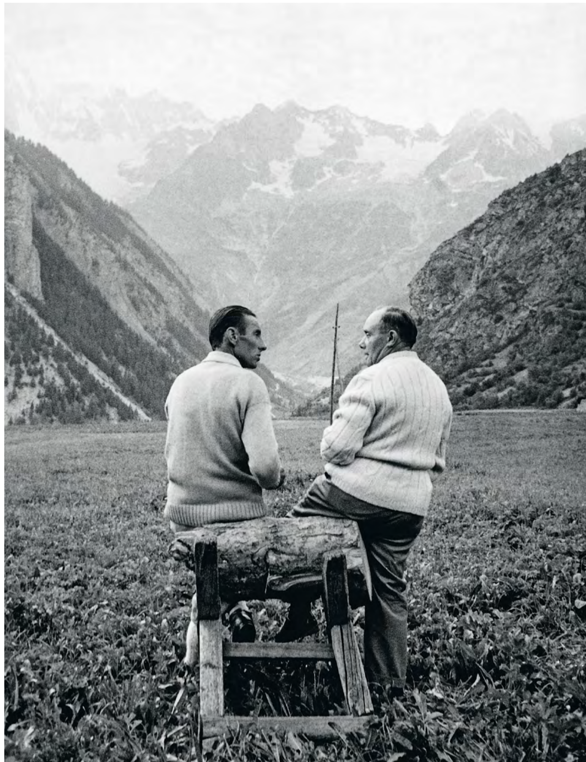
The Italian building surveyor Pietro Alaria discussing the construction works of the Mont Blanc Tunnel with the Alpine guide Ubaldo Rey. Valle d'Aosta, August 1962 ©Giorgio Lotri/Mondadori Portfolio via Getty Images
